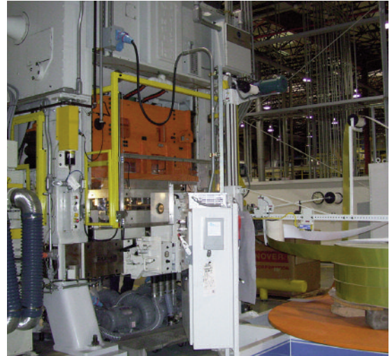
Power to the uncoiler in front of this Stolle Cupping System can be disconnected easily for die changing or maintenance, using the Meltric Deconnector visible above the die on the left side of the machine.
