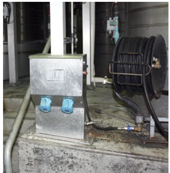
Meltric DECONTACTOR™ Series switch-rated Plugs and Receptacles provide a safe, quick and reliable way to connect and disconnect pumps, bottling machinery and harvest equipment to the 220V 3 phase outlets at ZD Wines.
